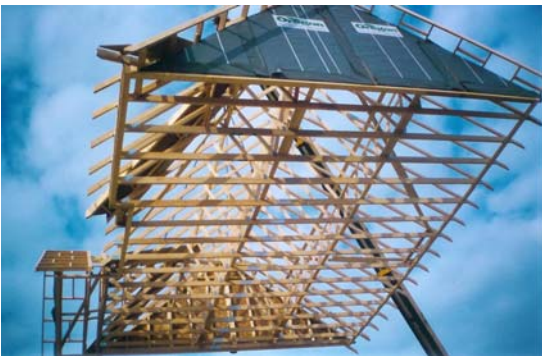
Figure 1 Crane erect of roof system
