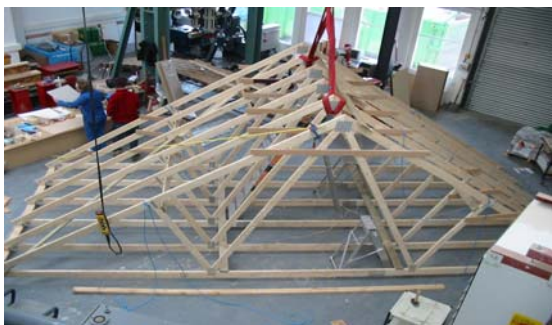
Figure 1 Crane erect of roof system
