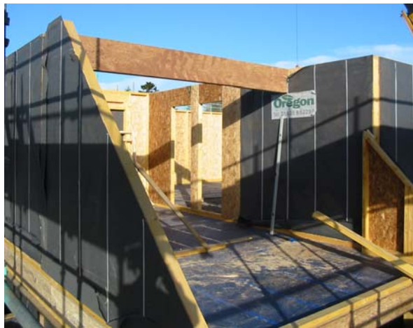
Figure 1 Timber platform frame during construction
